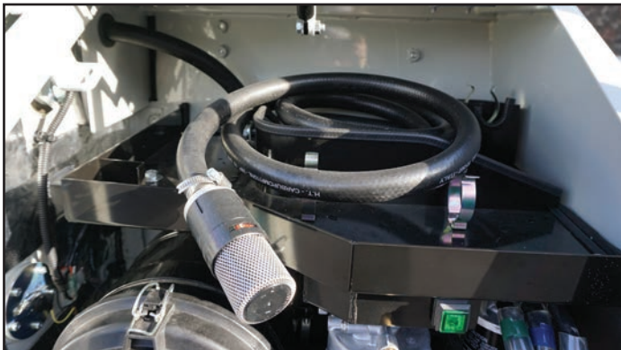
Fuel Transfer Pump
